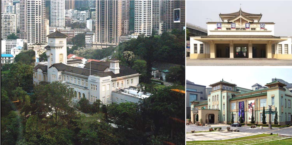
The current Government House (1944-today), designed by Japanese architect Kensuke Aiga of the South Manchurian Railway Company – 帝冠式様. Compared with Japanese colonial architecture in Taiwan: (top) Kaohsiung Train Station (1941) and Kaohsiung Museum of History (former government office) (1938).
