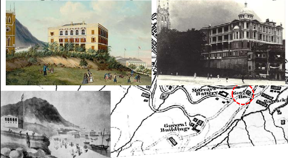
The second temporary Government House (1844-1846), later twice rebuilt on the same site, and much, much later adapted as the HKSAR Court of Final Appeal
