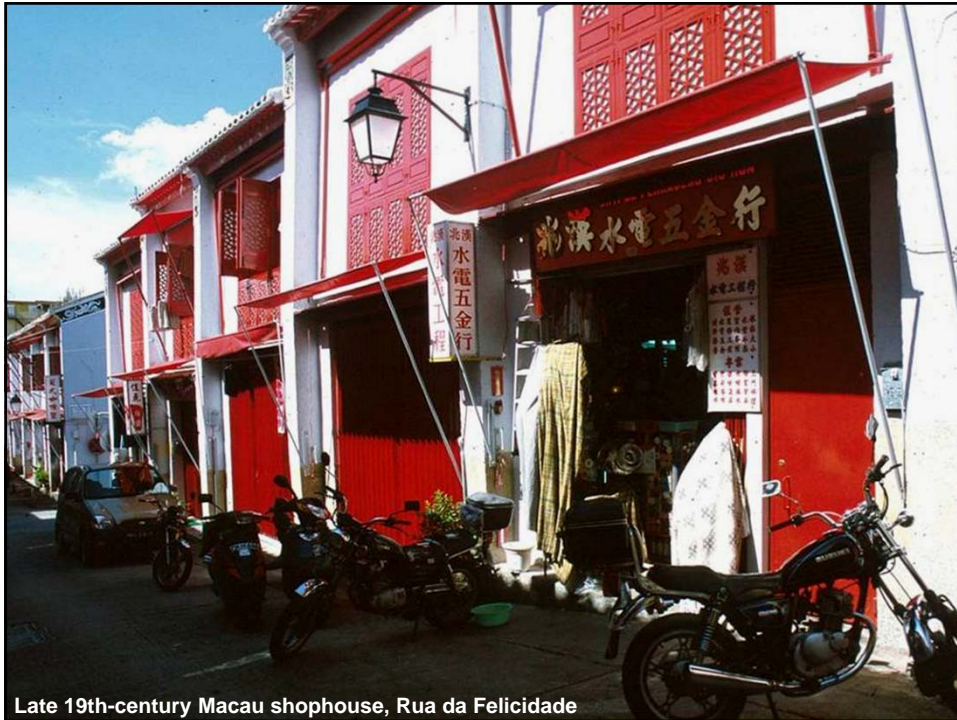
Late 19th-century Macau shophouse, Rua da Felicidade
