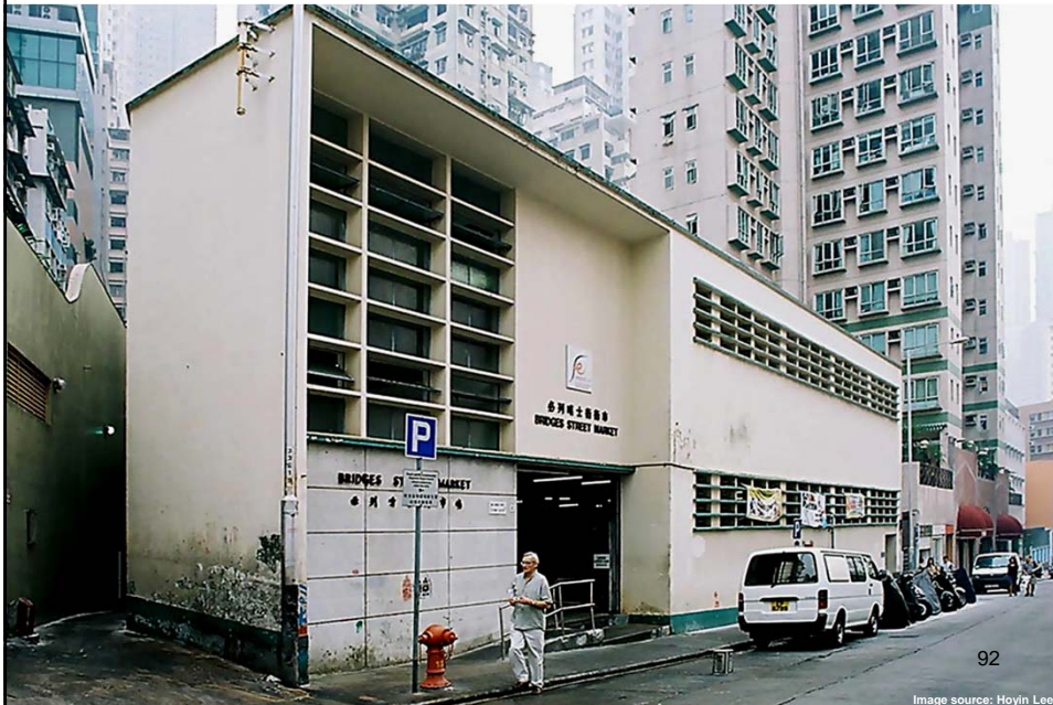
Bridges Street Market, Bridges Street, Hong Kong (1951)
