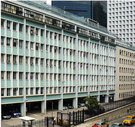
Central Government Offices West Wing, Hong Kong (1959)
