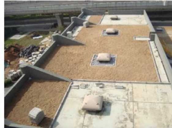
5. Placing planting soil
