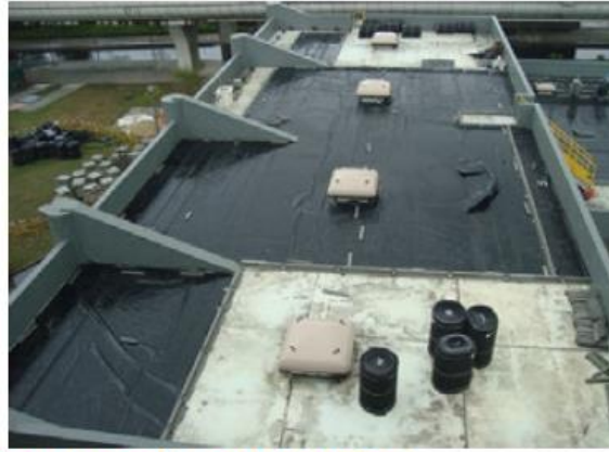
2. Install root barrier
