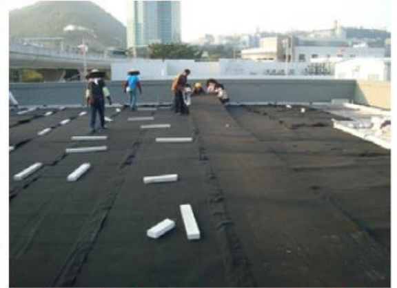
3. Install drainage composite layer
