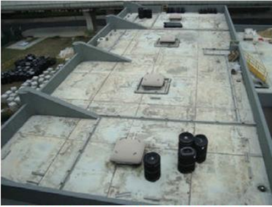
1. Clean up rooftop surface
