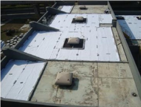
4. Install water retention mat
