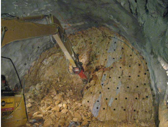
Cavern works by mechanical excavation 岩洞工程以機械挖掘方法施工
