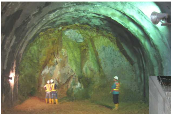
Geological mapping of rock face 為岩面進行地質測繪
